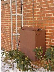
The Kenwood repeater is mounted vertically with the duplexer behind. Steve supplied these components, along with the antenna.
